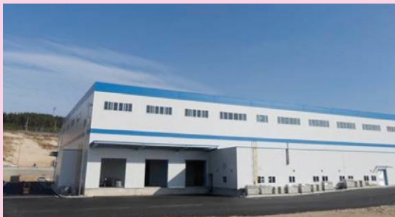
Figure 7 POSCO Power's stack manufacturing facility in Pohang, Korea
