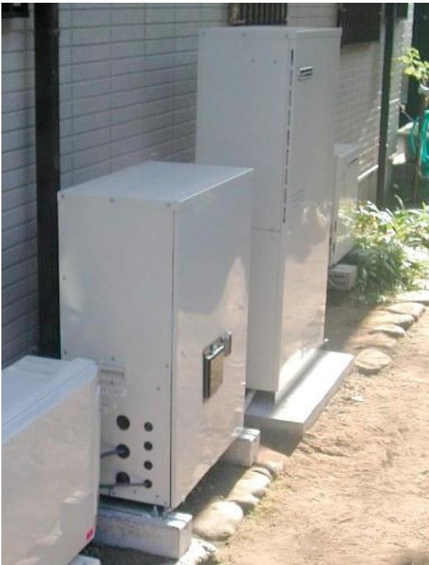
Figure 3: Toto SOFC, 0.7kW fuel cell unit on the left hand side, hot water tank unit on the right hand side.
