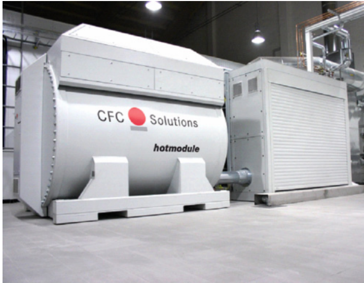
Figure 3. The “HotModule” system (courtesy of CFC)
