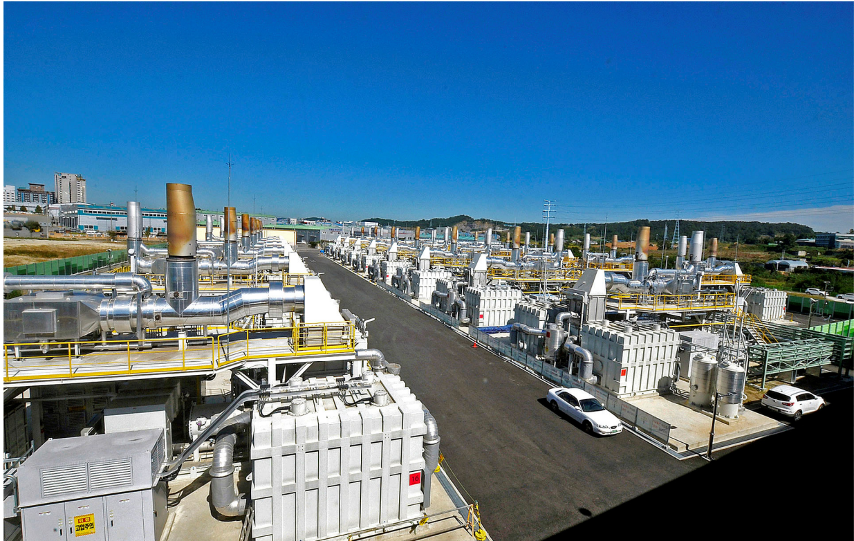
FIGURE 17 The world's largest fuel cell plant. 58.8 MW molten carbonate fuel cell park in Whasung City, Gyeonggi Province, South Korea (courtesy of FuelCell Energy Solutions)
