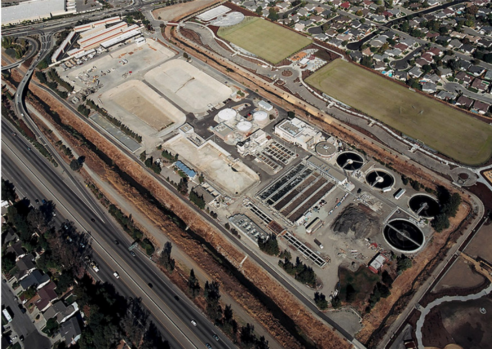
FIGURE 236 Dublin San Ramon wastewater treatment facility
